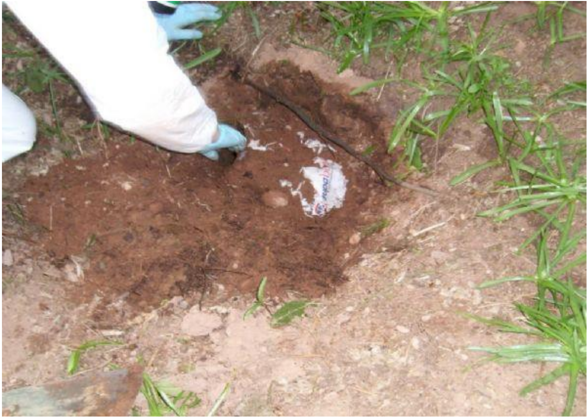
Sack being exposed
